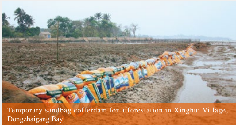
Temporary sandbag cofferdam for afforestation in Xinghui Village, Dongzhaigang Bay
