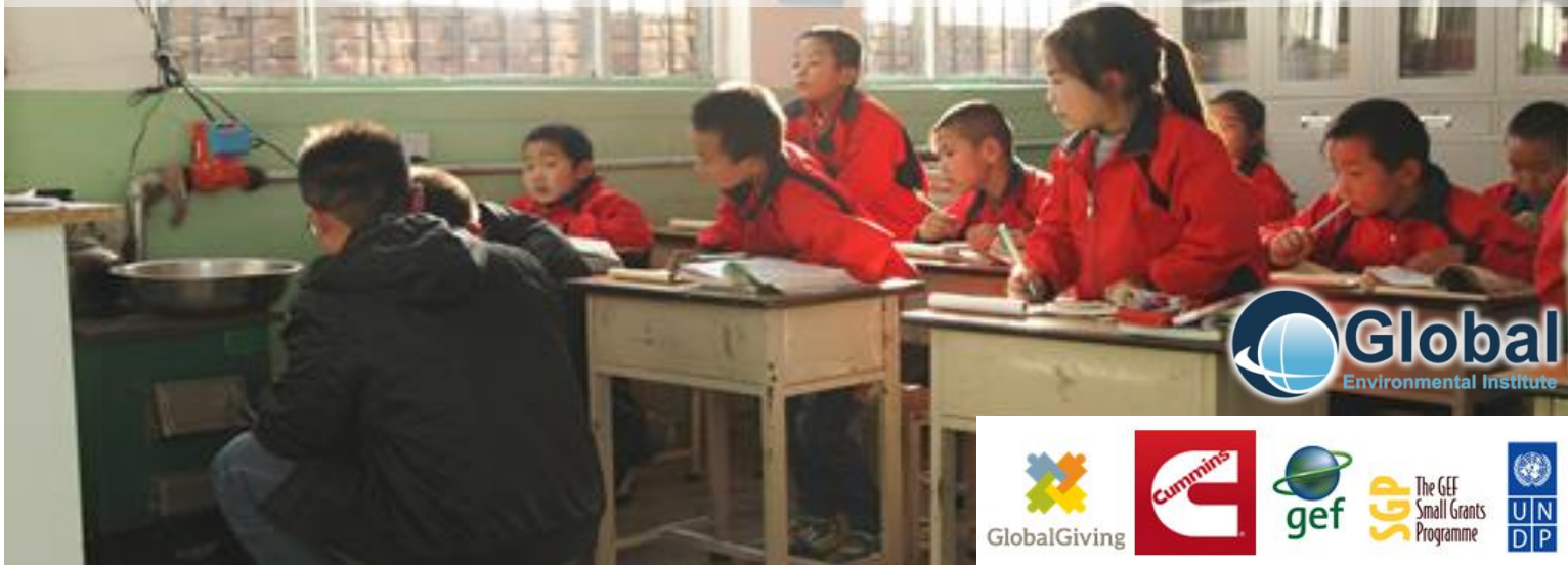
Schoolchildren look on as their classroom's new clean cook stove is installed – 2015 GEI
