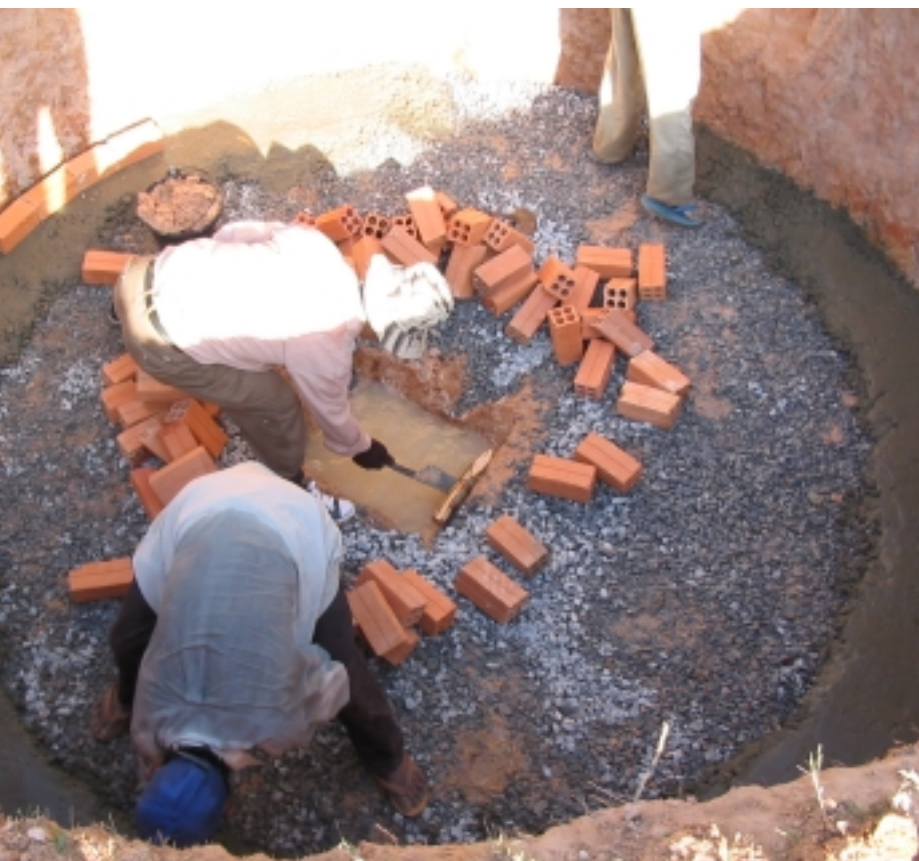
Figure 11 Constructing the Base
